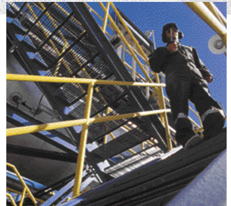
Technical potassium nitrate plant.
