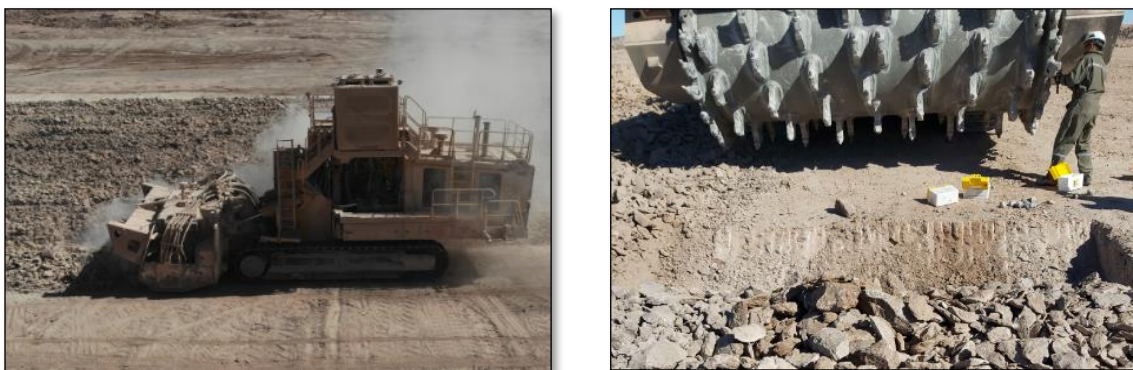
Figure 13-3. Terrain Leveler Surface Excavation Machine (SEM)
