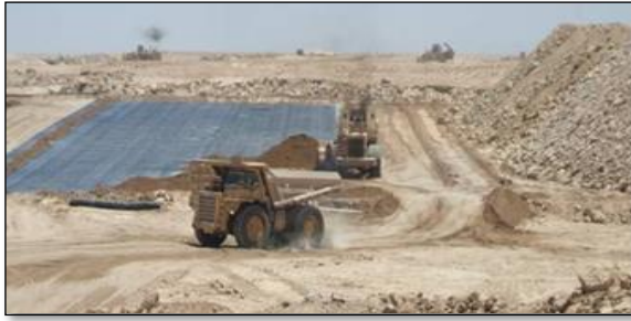
Figure 13-1. Pad Construction and morphology in Caliche Mines
