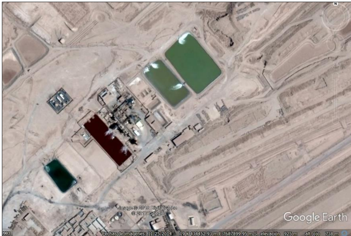
Figure 15-8. General View of the Iris Iodine Plant Area
