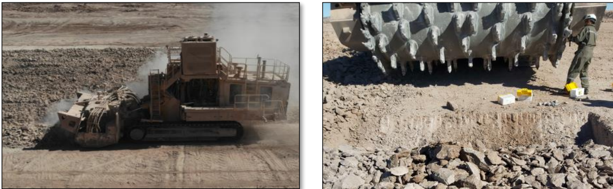
Figure 13-6. Terrain Leveler and SME equipment (Vermeer)
